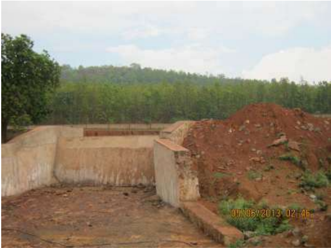
Fig. 5.6: Implemented Check Dam
