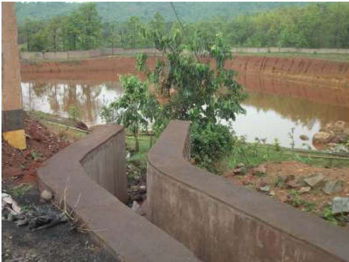
Fig. 5.7: Part of Implemented Drainage Network Connecting Reservoir
